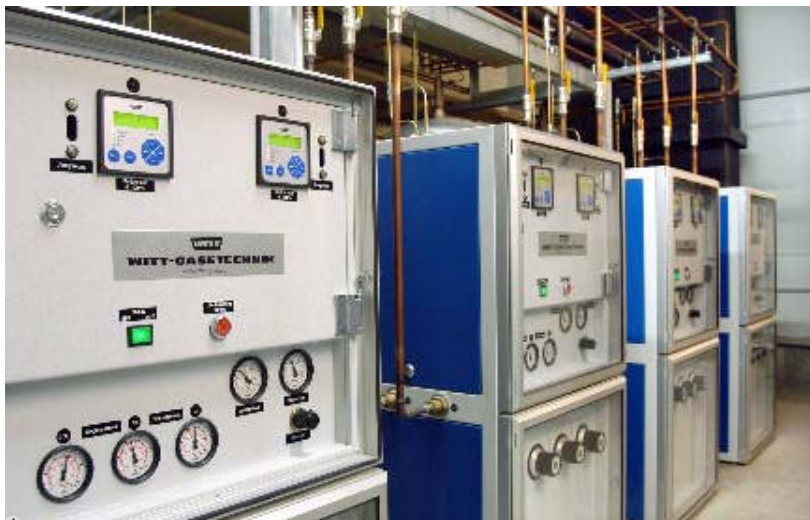
Centrale gas-supply for 22 packaging lines
